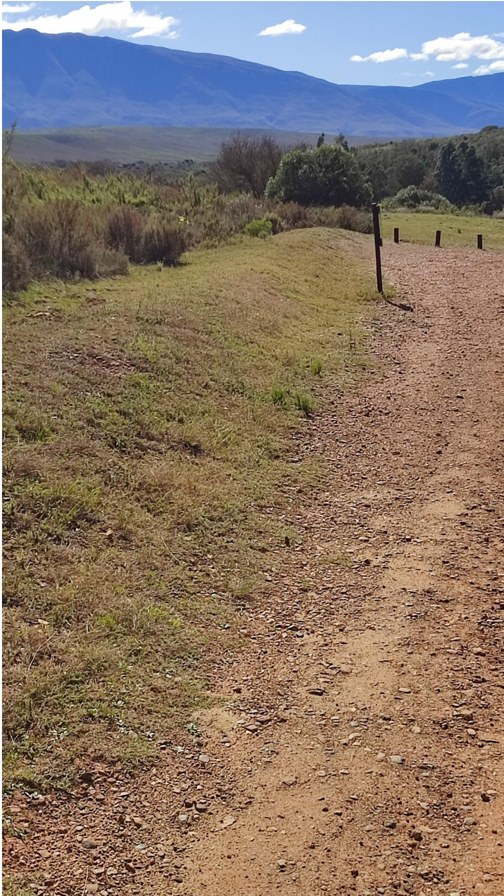
Photo 7: Area where pipelines to new soak away will be laid (Photo taken 17/08/2022)
