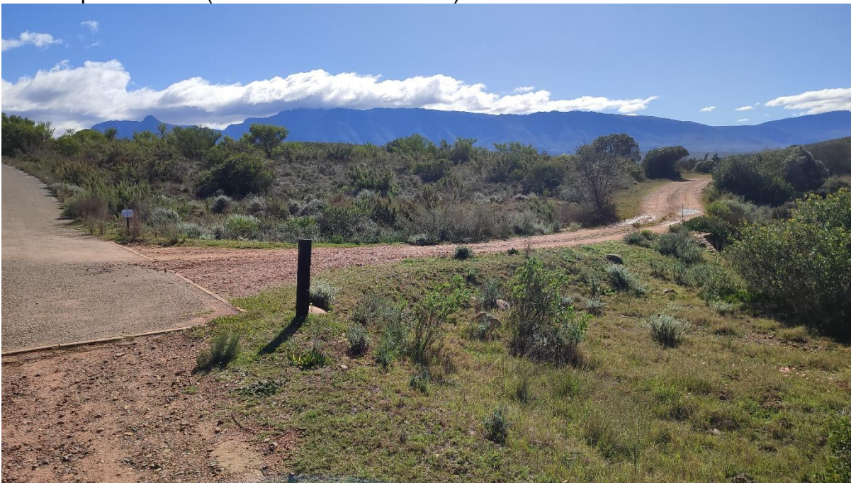
Photo 6: Existing road along which new pipelines and cable will be laid. (Photo taken 17/08/2022).
