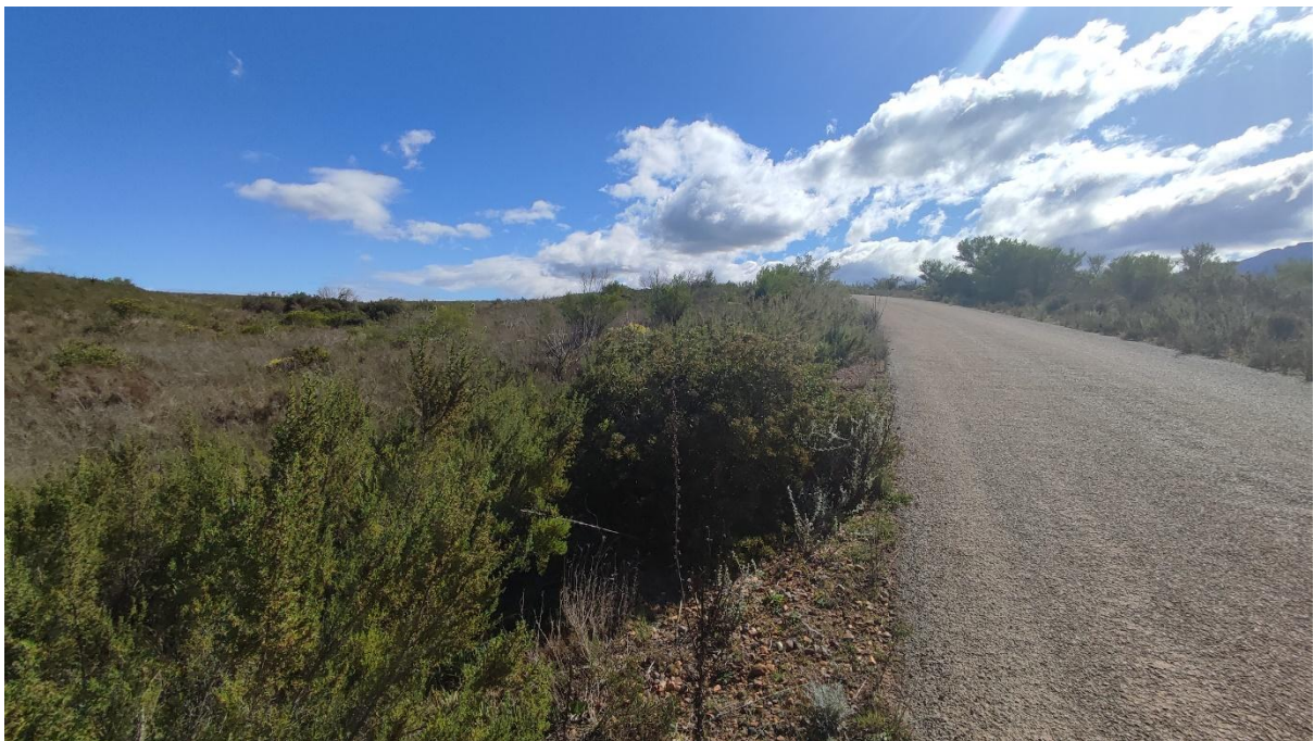
Photo 9: Access road to picnic site along which additional parking bays are proposed. (photo taken 17/08/2022)
