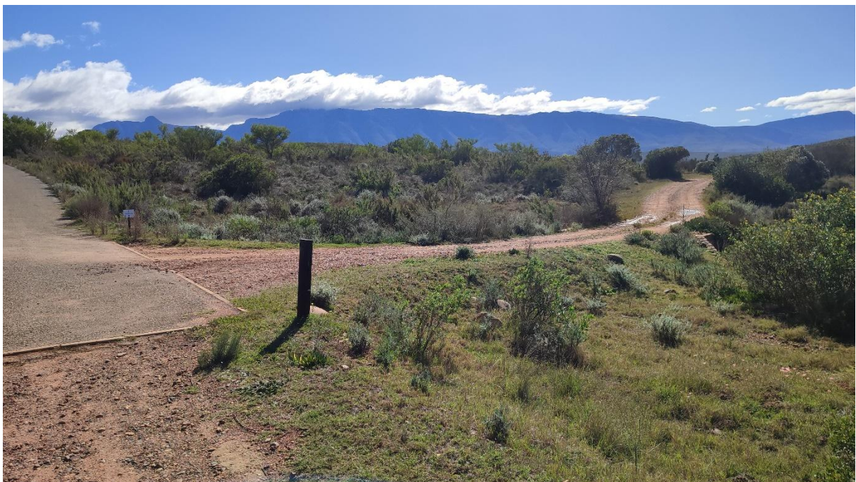
Photo 4: Existing road along which new pipelines and cable will be laid. (Photo taken 17/08/2022).
