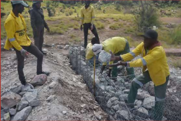
Mitigation work to control erosion of archaeological materials in Mapungubwe National Park include left, a retaining wall at K2 and right, erosion containment at Schroda.
