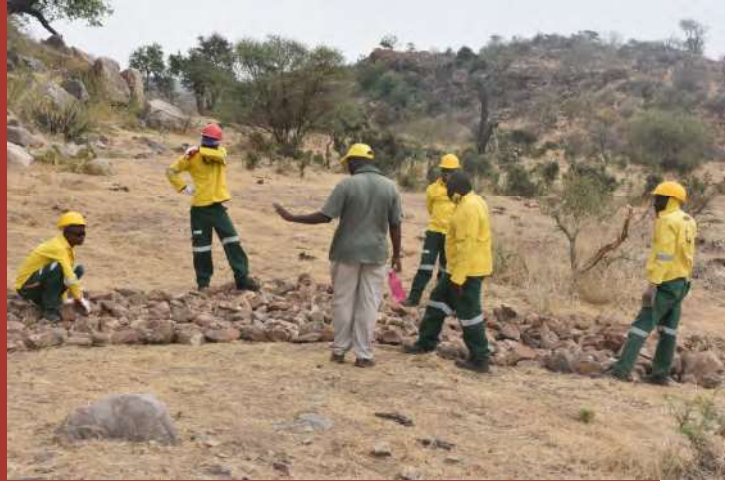
Mitigation work to control erosion of archaeological materials in Mapungubwe National Park include left, a retaining wall at K2 and right, erosion containment at Schroda.
