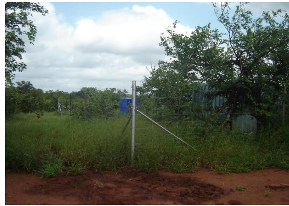
The construction area is temporary fenced.
