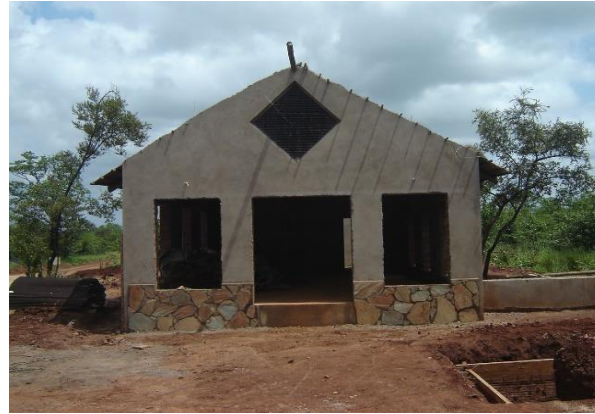
The contractor is busy with the construction of the buildings.
