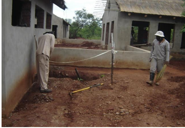
Concrete is mixed on impermeable surface.
