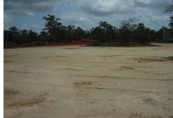
The parking area is cleared.
