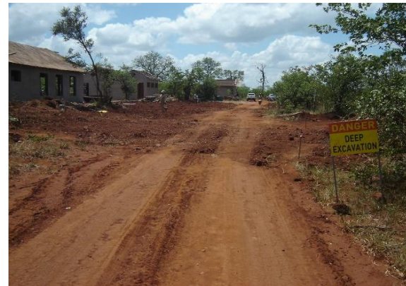
Existing access road is use for acces to the construction site.
