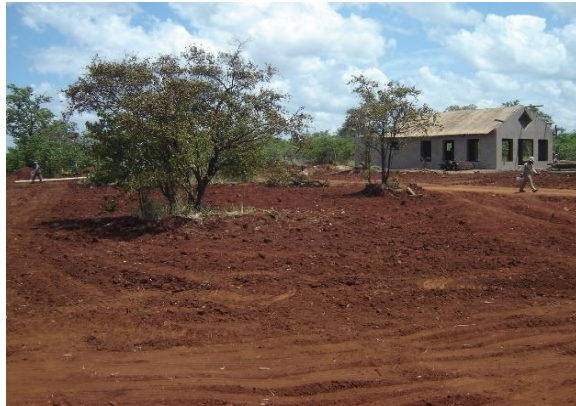
The parking area is cleared.
