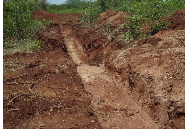
Trenches for the sewer pipeline.
