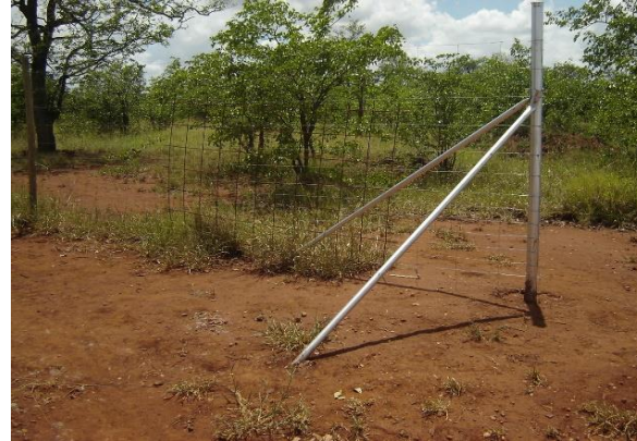
The construction area is temporary fenced.
