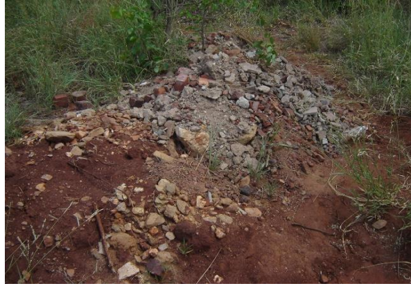
Concrete is mixed on impermeable surface.
