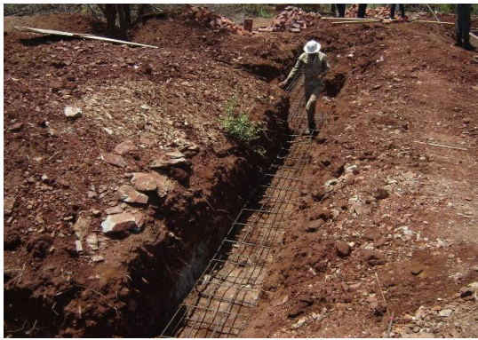
The foundations are excavated.
