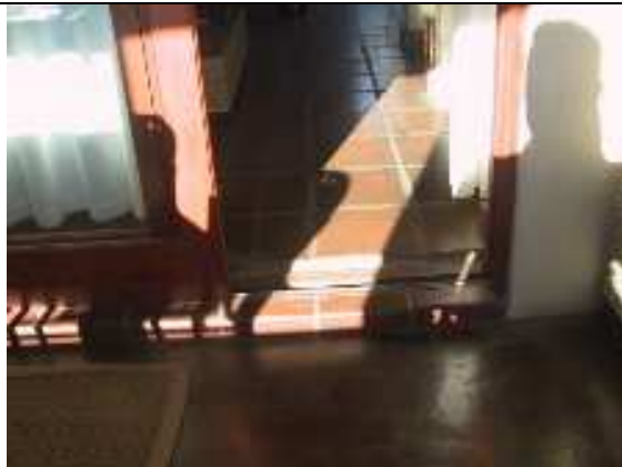
Step from veranda into TV Room/Kitchen Area
