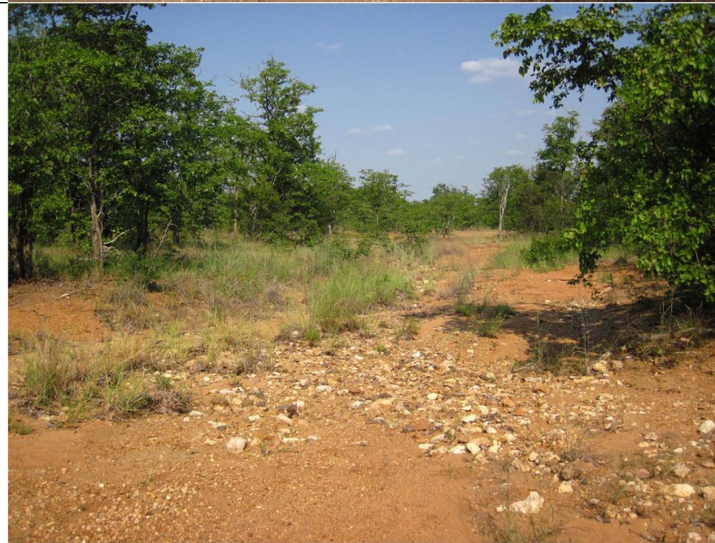
Photo 14: One of many storm water drainage lines along the Shangoni Ranger road to be upgraded
