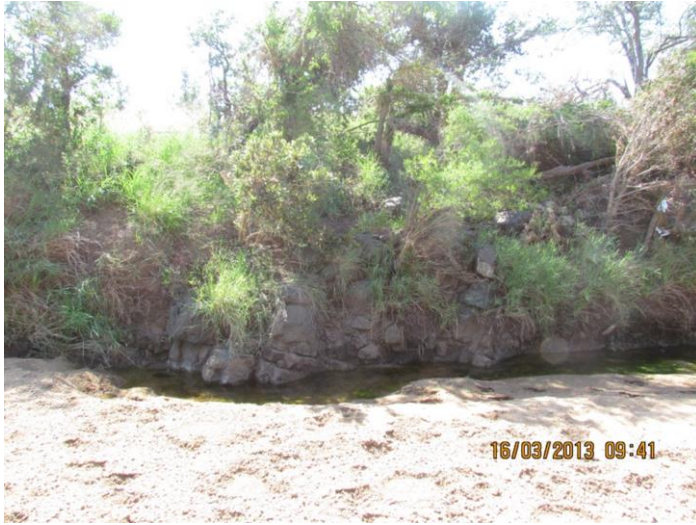
Dolorite outcrop on left hand embankment of river at proposed bridge location
