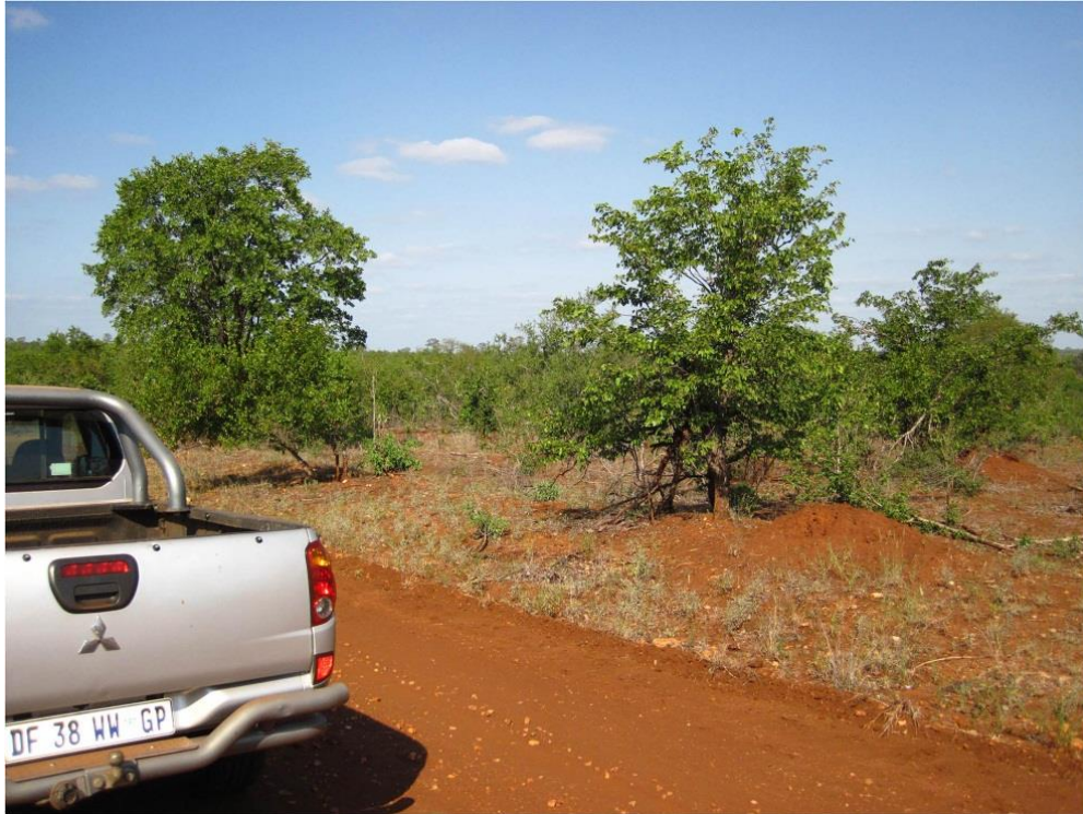
Figure 10: The eastern position of the new alignment where it will join the Shangoni Patrol Road at 23° 09' 45.2"S; 30° 52' 20.6"E.
