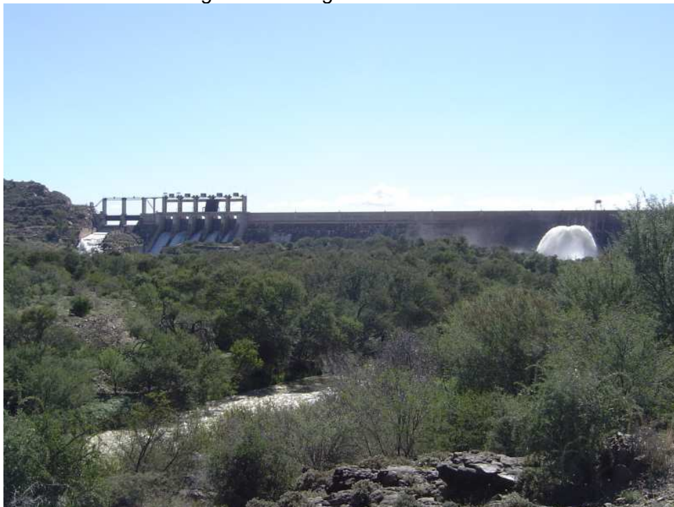
Figure 6: View towards dam wall from low level bridge (concession starting point)
