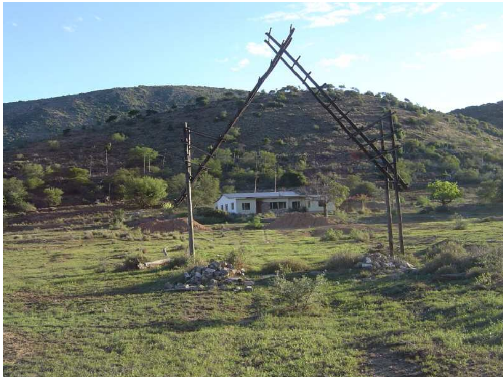
Figure 16: Pietersenskraal (requires refurbishing)
