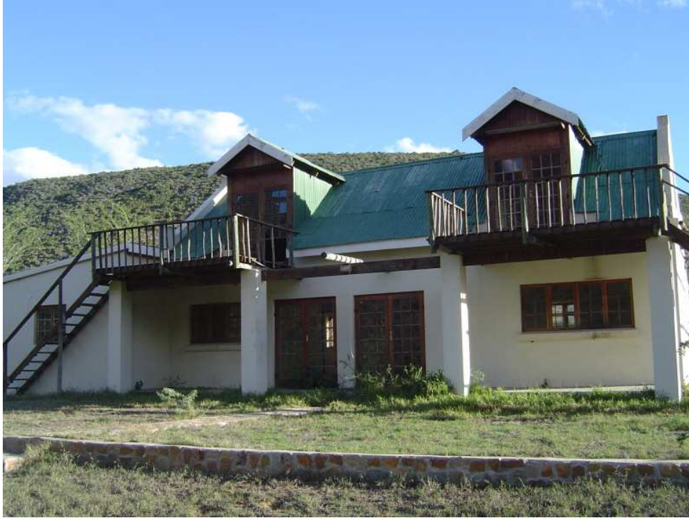
Figure 11: River Lodge (Requires major Refurbishing)
