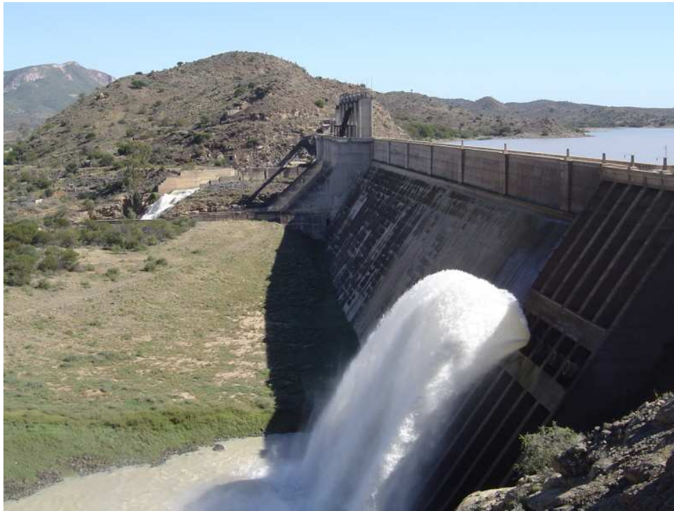
Figure 5: Darlington Lake Dam wall
