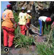
4 Packing and laying stone
