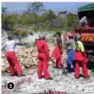
2-3 Transporting stone to site
