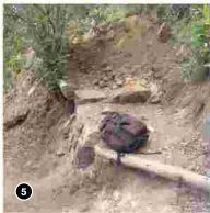
7-8 Dry packed stones stabilise path; Newlands Forest
