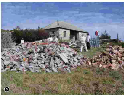
1-5: Renovating the Overseers Cottage, Eastern Back Table
